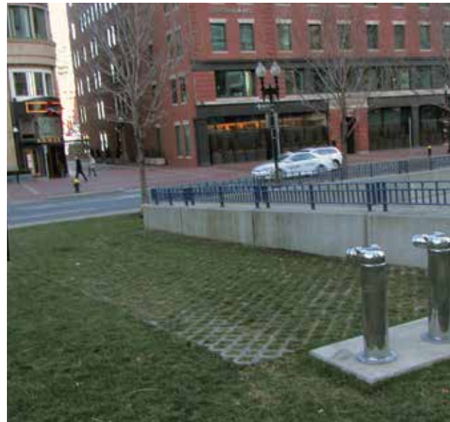
Figure 13. Concrete grid pavement typically reduces runoff in a manner similar to grassed surfaces.
