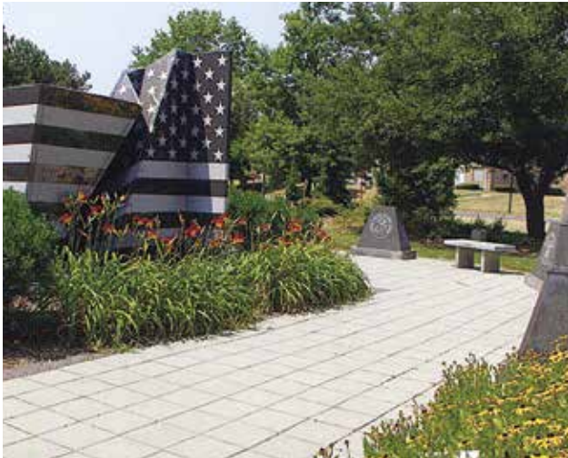
Figure 14. High SR paving slabs
